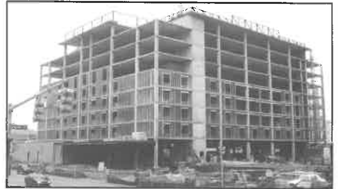
Charleston's New $26 Million Embassy Suites Hotel Now Under Construction
