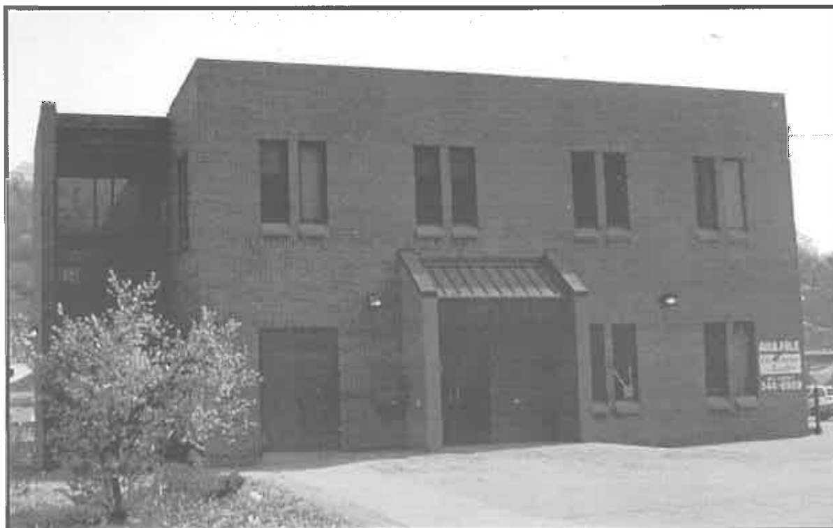
This East End office building is the future home of ACT and the State Building Trades
