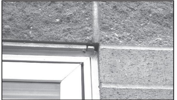
THIS PICTURE SHOWS a lentils that is too short. It was installed by Lang Masonry and is just one of many examples of shoddy work found and documented at the Frontier High School.
