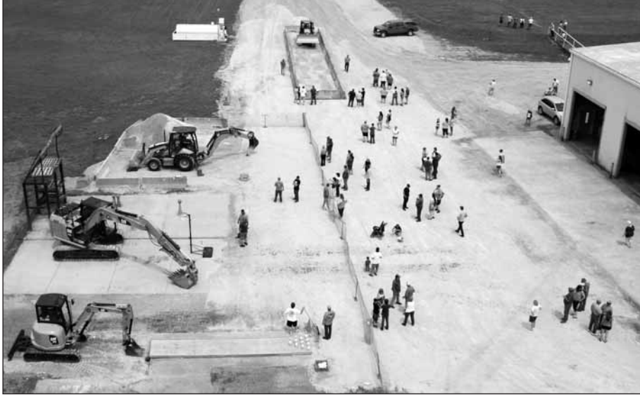
This shot, taken from the tower crane on the Operating Engineers Local 132 training site in Medina, shows the set up for the equipment rodeo event held in mid-June.
