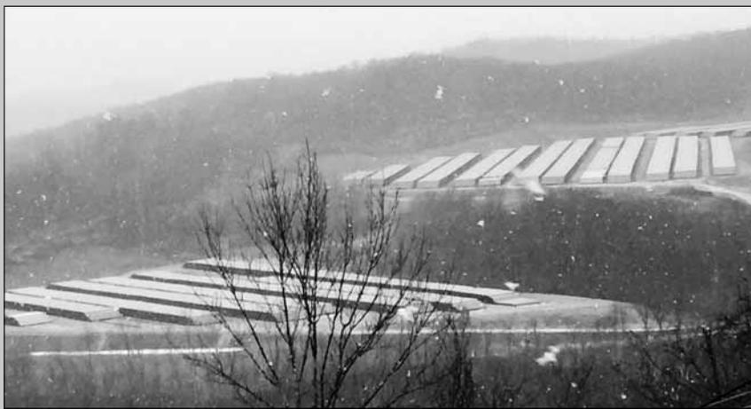
Miles of pipe wait to be turned into the Atlantic Coast Pipeline by union workers. The stockpile is in the Morgantown area. The pipe pictured is 42 inches in diameter.
