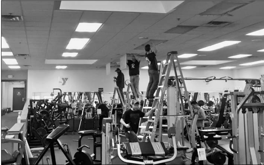
Members of IBEW Local 968 Parkersburg (on ladders from left) Rocky Griffin, Dave Lamp Jr., Ethan Mills and Levi Mills (standing) help replace light fixtures at the Parkersburg YMCA. Other members who volunteered were Dakota Hunt, Brye Mullenix, Jarred Smith, Lorne Mills, Chris Smith, Lyn Lovell, and Clayton Griffin.
